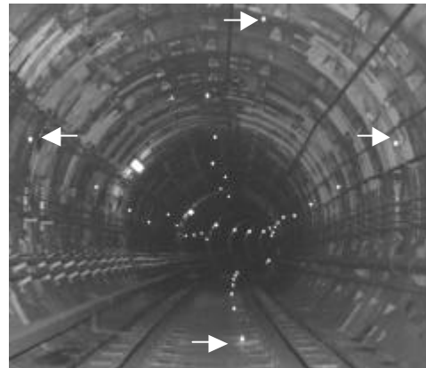
Fig. 6 Picture of Tunnel with prisms
